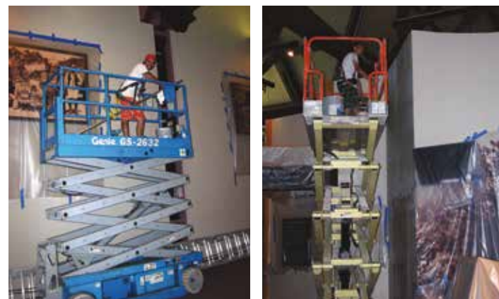
Contract workers scale the heights to clean and paint the Museum ceiling.
