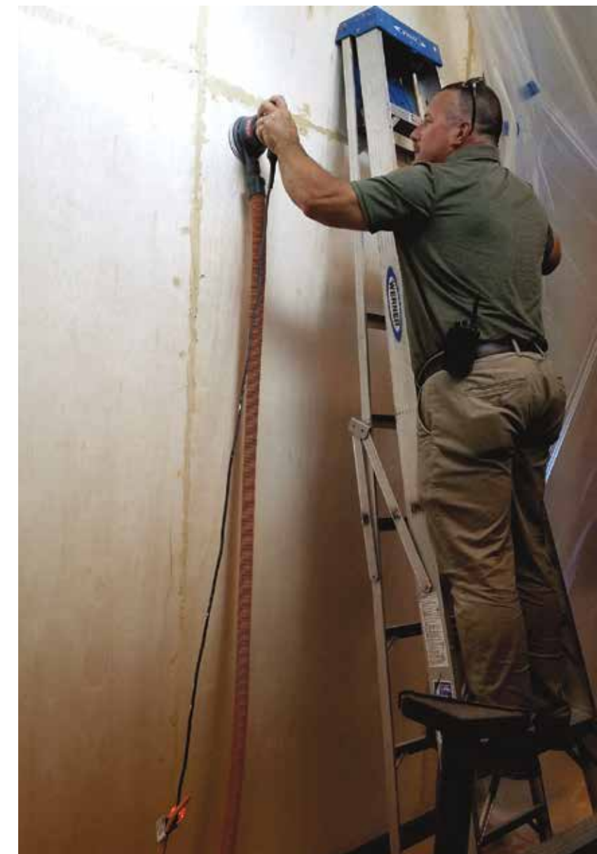
Facilities Manager David Higgins works on the new wall in the Mosaic Community Art Gallery.
