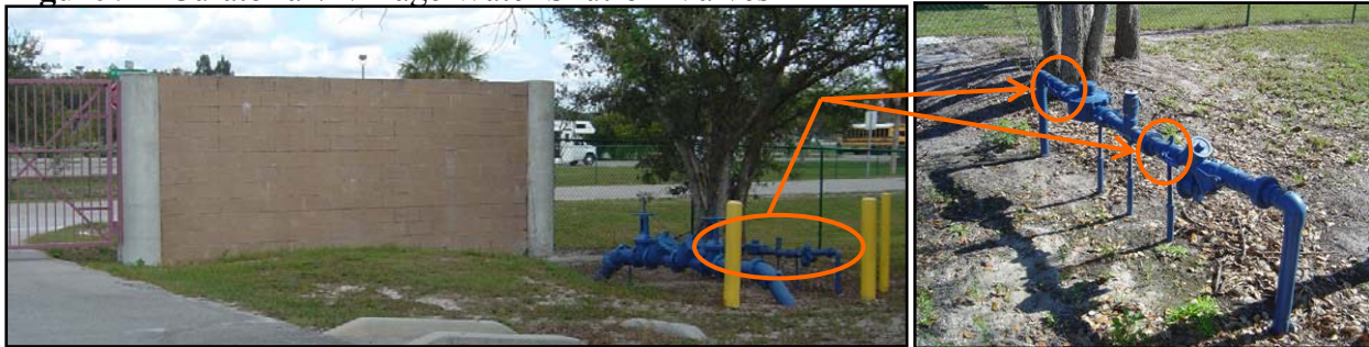
Figure 9 – Curatorial / Village Water Shut-off Valves
